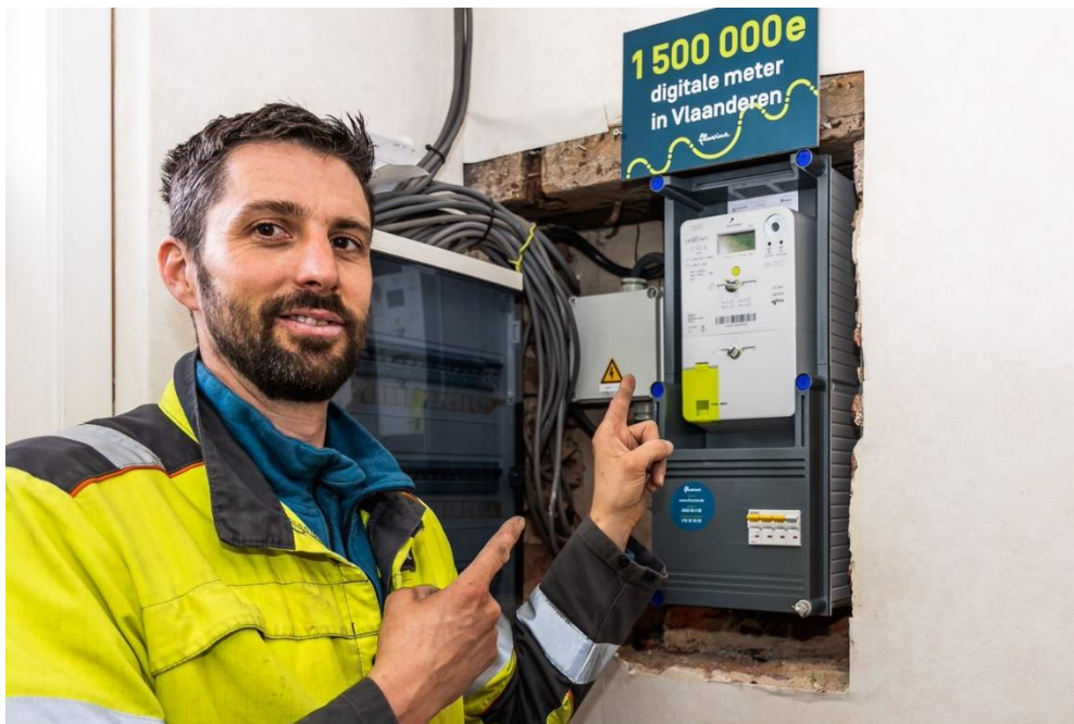
Already 1,5 million digital meters installed
