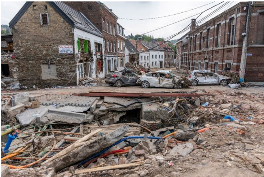
Enormous damage after the floodings
