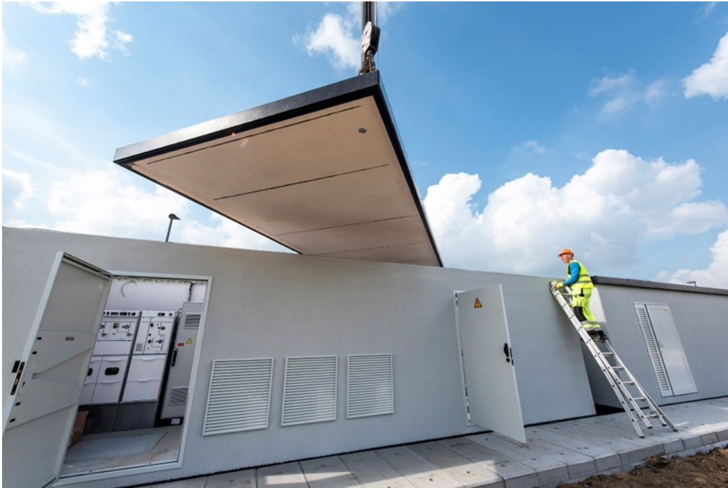
Installation of a cabin at the Green Energy Park (Zellik)
